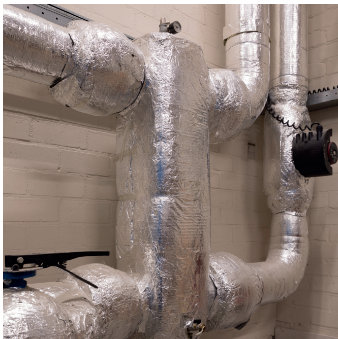
Isolation around heating pipes
